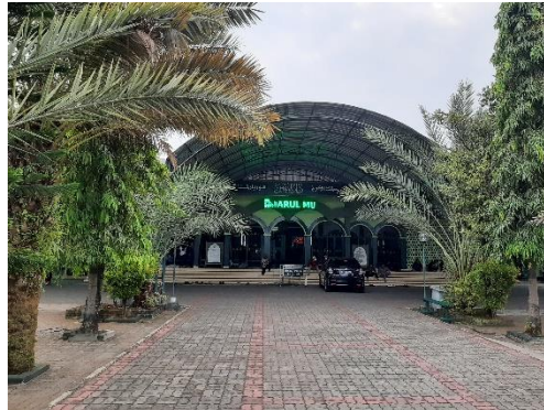
Figure 6. Tarpaulin in Jami' Darul Mutaqqim Mosque
