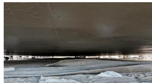
Gambar 1. Flat bottom finish coating
