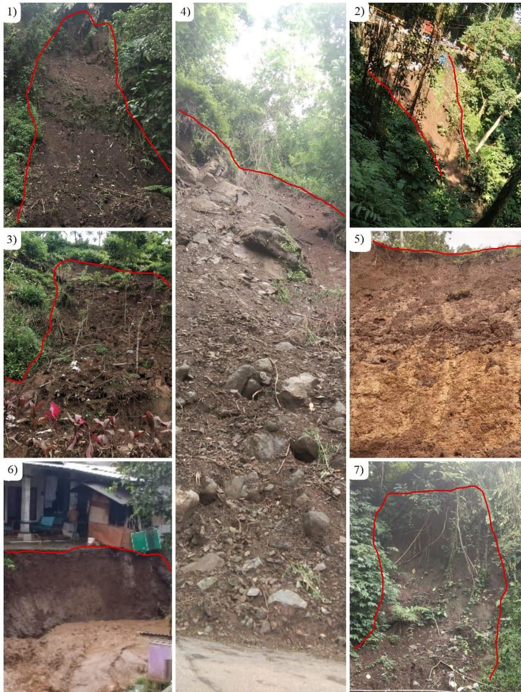
Gambar 10. Tipe Longsoran: (1) *Planar Slide*; (2) *Slide Flow*; (3) *Rotasional Slide*; (4) *Rock fall*; (5) *Rotasional Slide*; (6) *Rotasional Slide*; (7) *Rotasional Slide*
