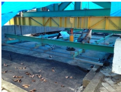
Figure 3 Loading test on the edge of slab
