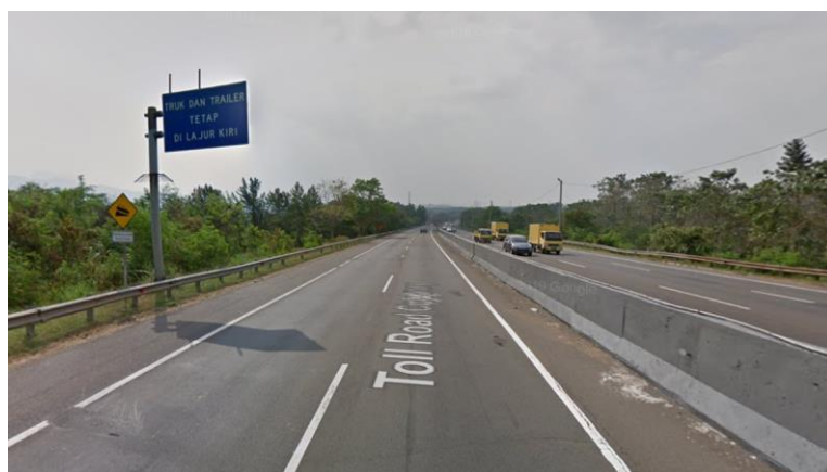
Figure 3. Warning sign of the downhill at Cipularang toll road
