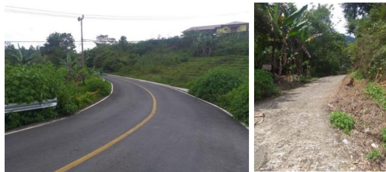
Figure 3. Road Network Condition in Tuktuk Siadong Village
